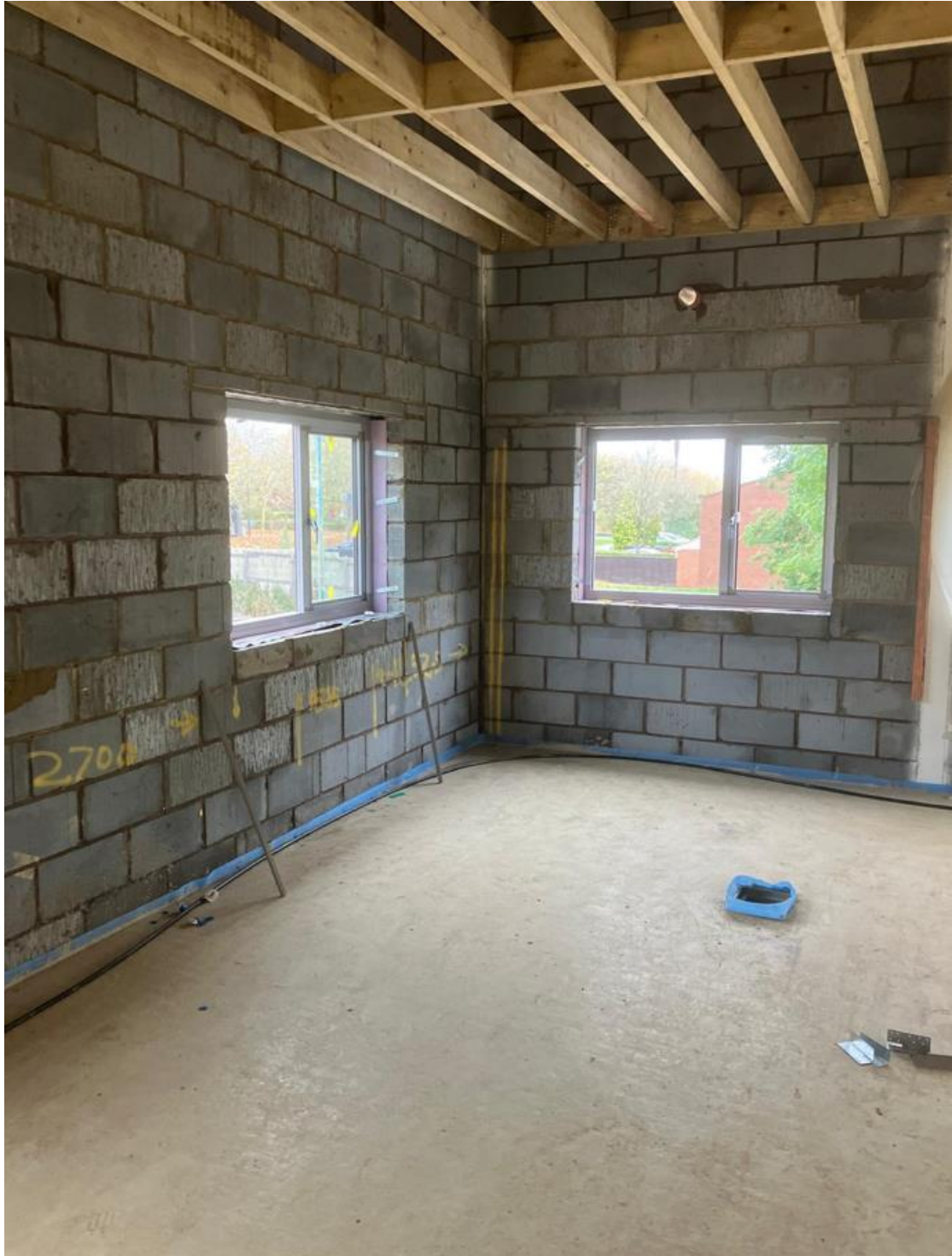
Ceiling Joists Installed to 1 st Floor.
