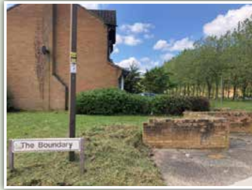
Photo after the work has been completed
