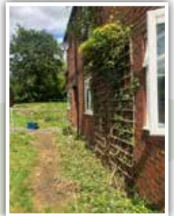
Photo after the work had been done
